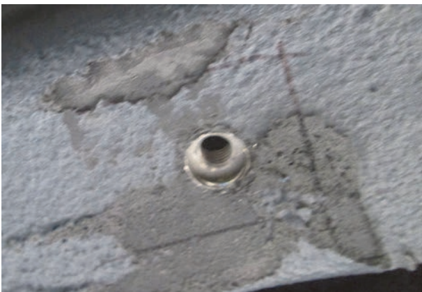
Figure 11: Hole with Anchorage Plate
