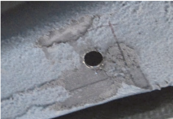
Figure 10: Member Fastening Holes
